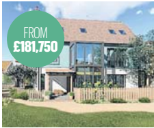
ESSEX Designed to Passivhaus principles around greens with fruit trees, the 51 rural custom-build homes at Oakley Orchards are 10 miles from Manningtree. Layouts vary from two to five bedrooms. 01803 814076, oakleyorchards.com
