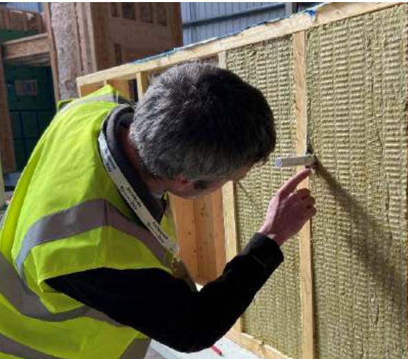
Coaction/BE-ST contractor training
