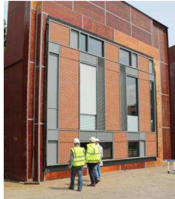
Inspection of the façade mock-up prior to air & water testing at Wind-techs Telford Facility. Colours and workmanship benchmark.
