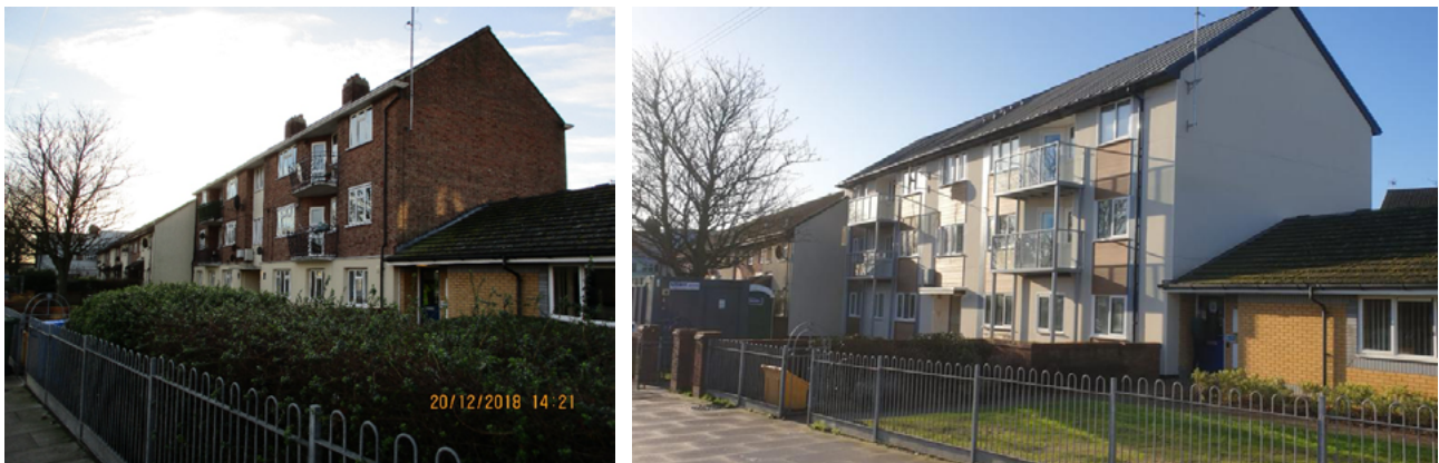
Above: Certified EnerPHit at King Street, Great Yarmouth - before and after
