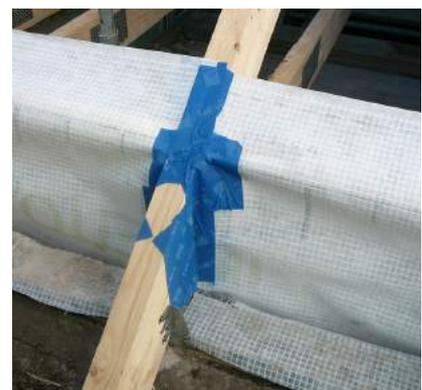
**Figure 21** Photo of airtight membrane connecting internal air barrier to membrane over the roof joists
