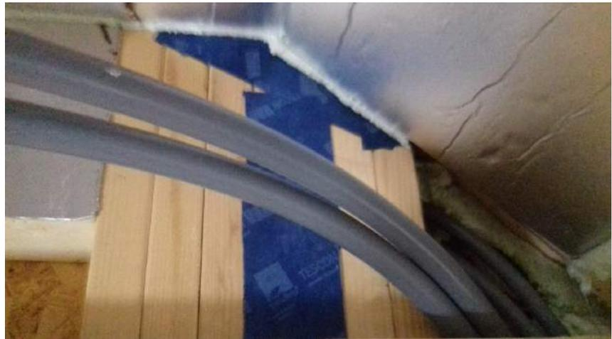
**Figure 30** Multiple timber posts penetration roof air barrier
