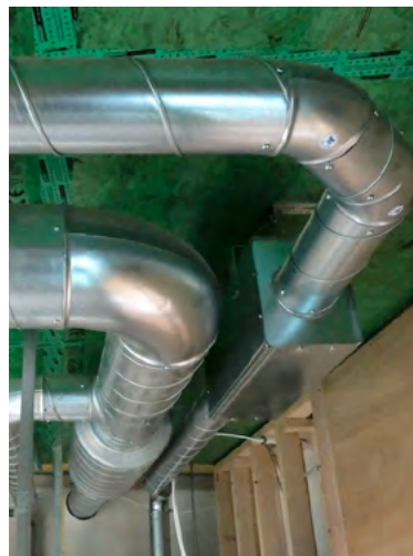
Rigid steel (left) and semi-rigid (right) ductwork. Images: Walled Garden, Nigel Dutt (l); New Forest EnerPHit, Ruth Butler (r)
