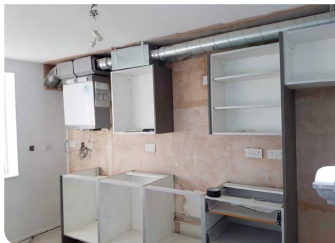
Below: small MVHR unit (on the far left) and ductwork discreetly built into and over kitchen cupboards.
