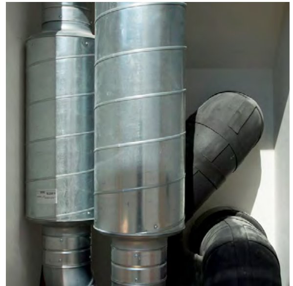
Circular silencers. Image: Earthwise Construction
