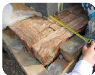
Check construction tolerances. Insulation is encapsulated tightly between internal and external leaf to avoid thermal bypass.
