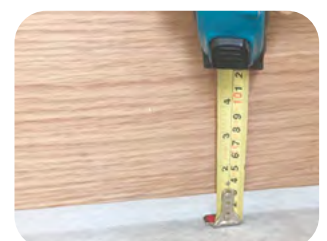
Air transfer provision is checked against design drawings and specification.
