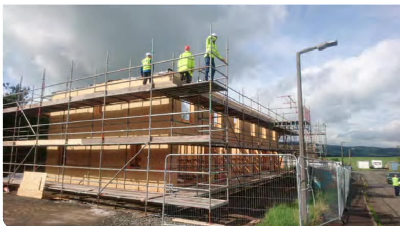
Below: under construction. Image: John Gilbert Architects
