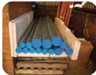
Ductwork protected from site debris during storage.
