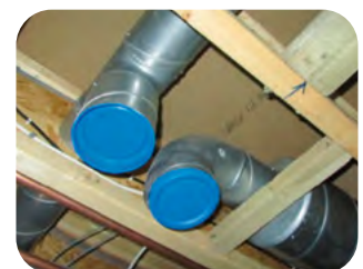
Ductwork protected from site debris during installation.
